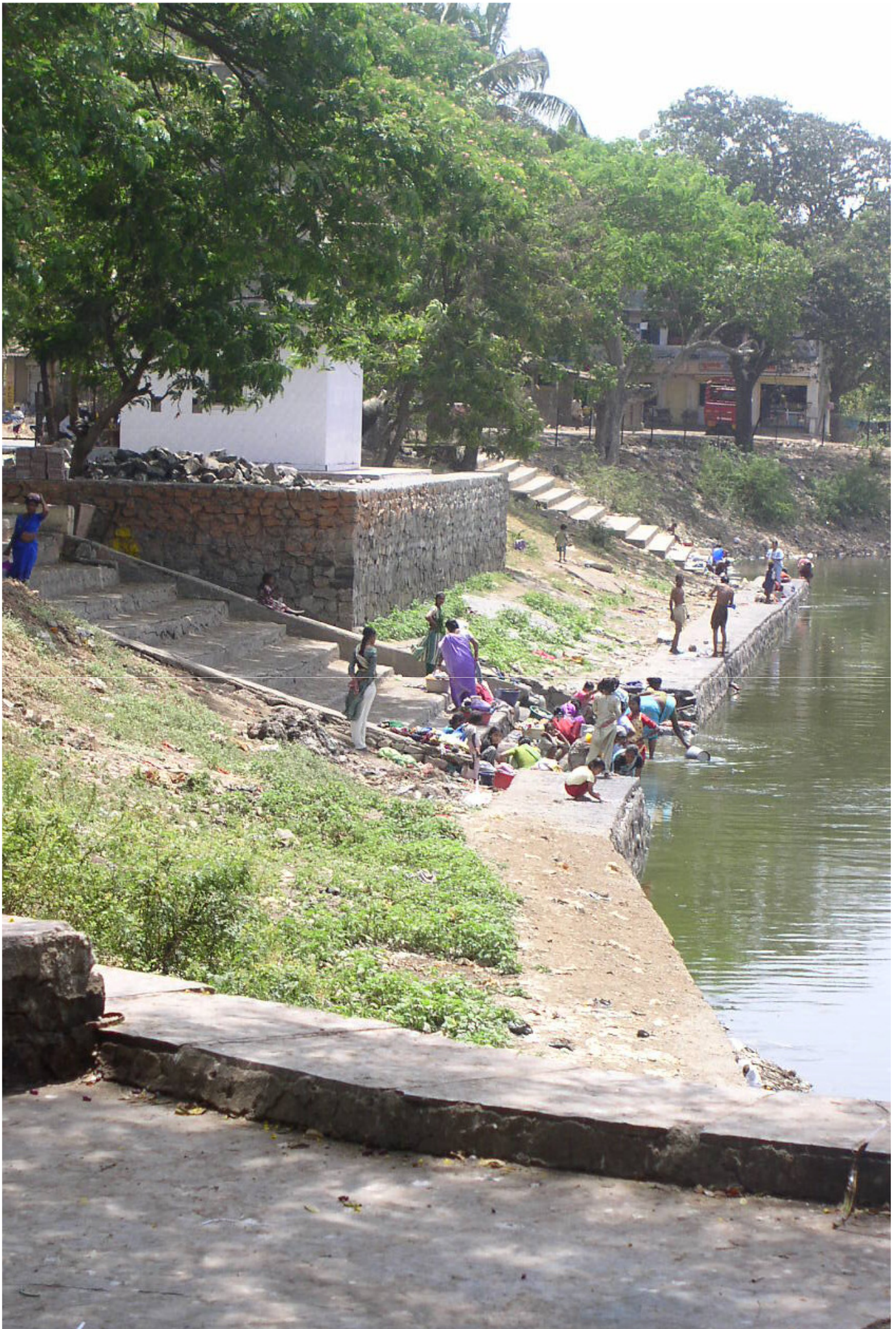
Newly constructed ghats along the edge
