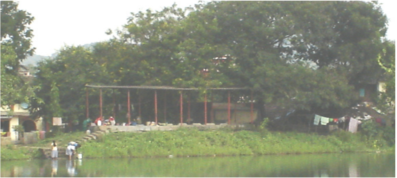
Washing shed along the longer edge which prevents waste water from entering the talav
