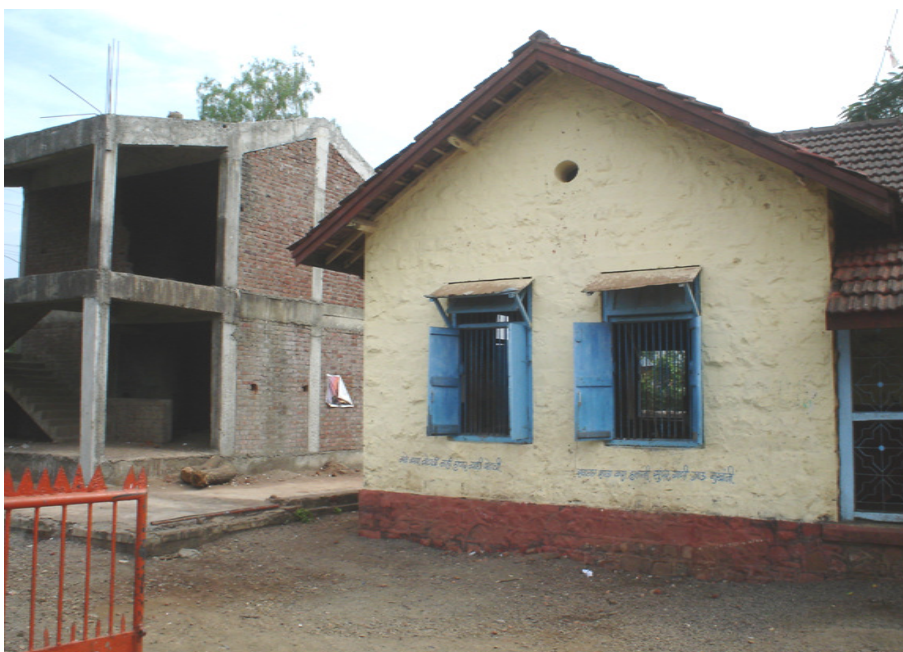
Extension to the school building
