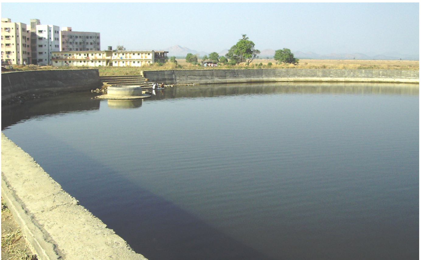
Recently constructed retaining wall in the foreground and new apartment buildings and transit camps in the background
