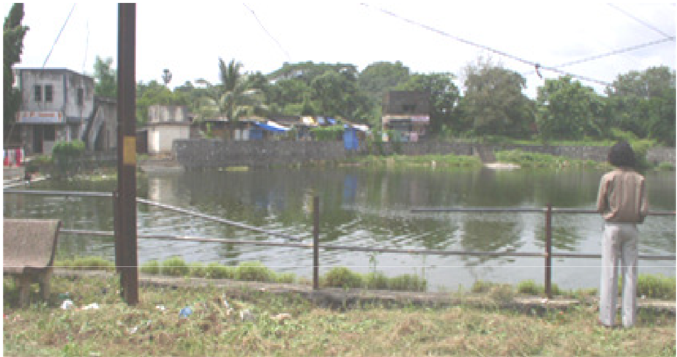
Transforming gaothan along the edge of the talav
