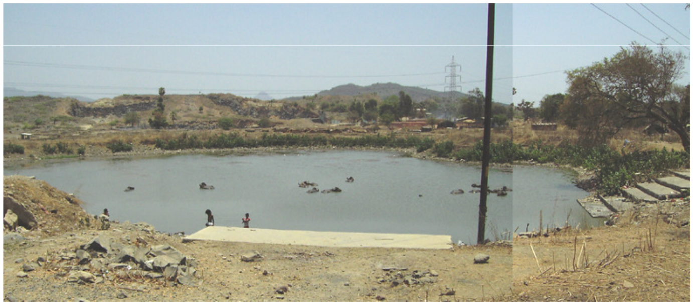
A washing platform and steps leading to the water form the chief architectural characteristics
