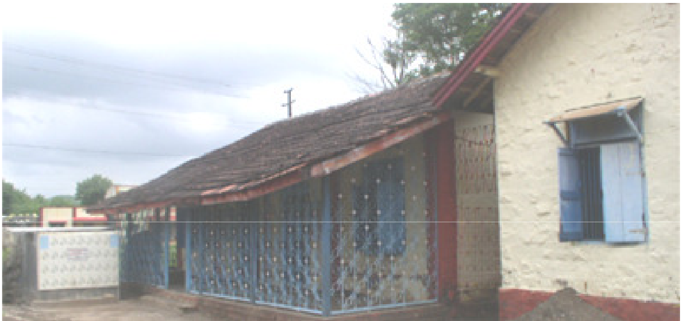
The school building with the verandah and the mangalore tile roof forms a background to the courtyard
